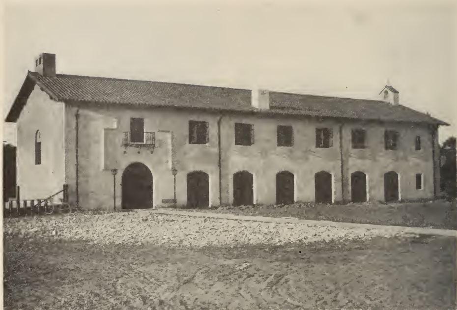
CATHEDRAL HOUSE, PHOENIX
